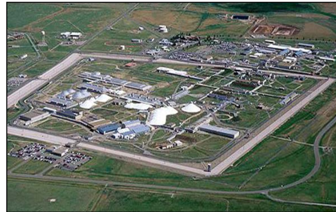
Inspect additional facilities
